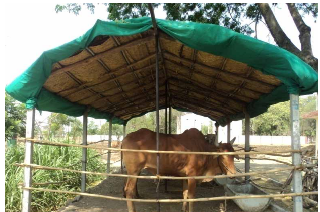
Loose Housing Cattle Barn
