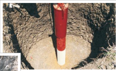
← Filling with filter material
