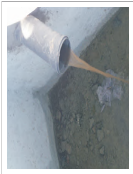
Runoff Water in Filtration Tank
