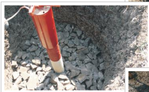
← Filling with filter material
