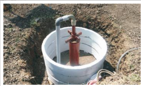
Laying of cement rings →
