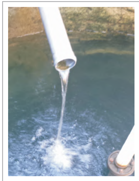
Filtered Water in Well
